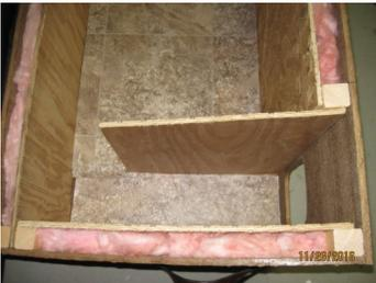
A view of the interior of the Alley Cat winter cat shelter plan displaying double insulated walls, insulation under vinyl flooring and wind guard.
