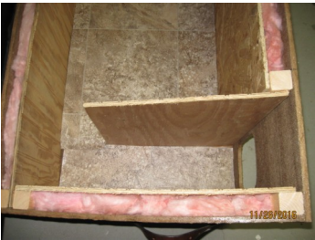
A view of the interior of the Alley Cat winter cat shelter plan displaying double insulated walls, insulation under vinyl flooring and wind guard.
